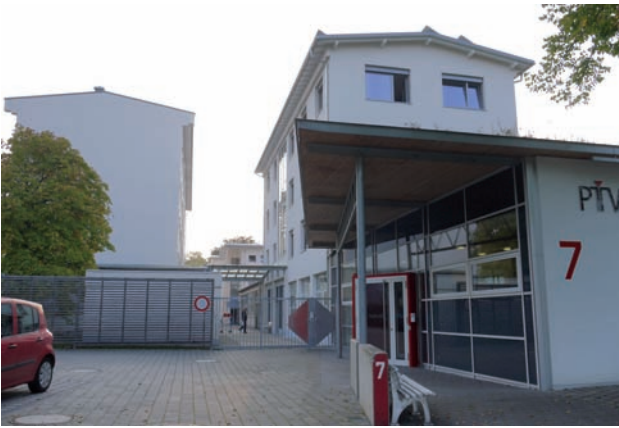
Front view of the PTW-Freiburg factory, building with calibration laboratory to the left. Chamber assembly building in the background
